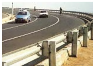
Road Safety Systems
